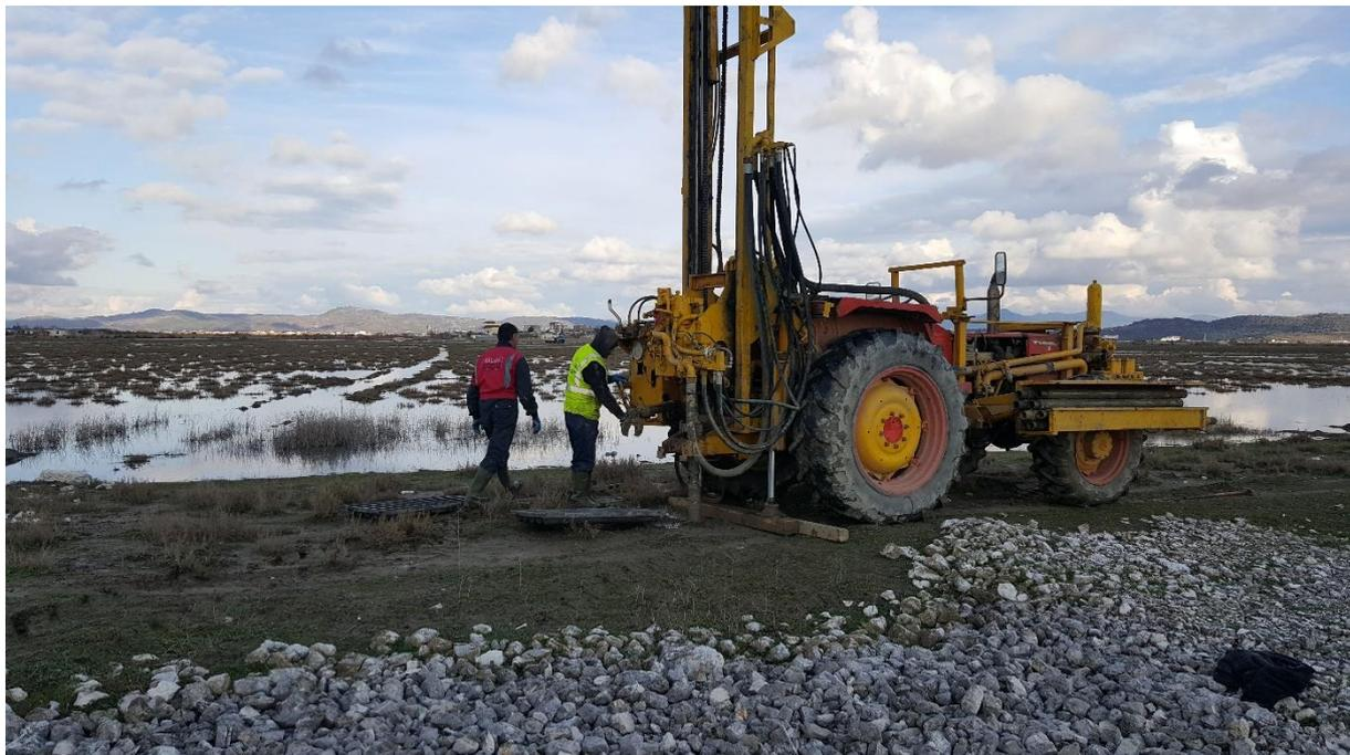
Figure 47- Photo while drilling, BH. Nr.2
